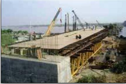
Figure 1: Superstructure Formwork Preparation
